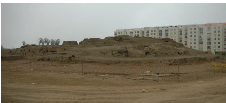
Figure 8: Huaca Huantinamarca (pre-Hispanic archaeological site located in the district of San Miguel, province of Lima, Peru) before the intervention. Source: (Santamaria, Bambarén, & Arias).
